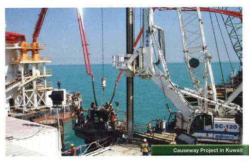
(sub-contractor for this project) about 760 piles given by two main contractors: 540 piles by **Hyundai Engineering & Construction Co. Ltd.**, and 220 piles by **Combine group Contracting Co**.
