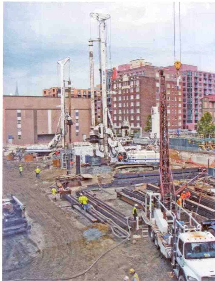
Each drilled shaft generates about 100 cubic yards of spoil that is dried using a hot lime mixture and then transported offsite.
