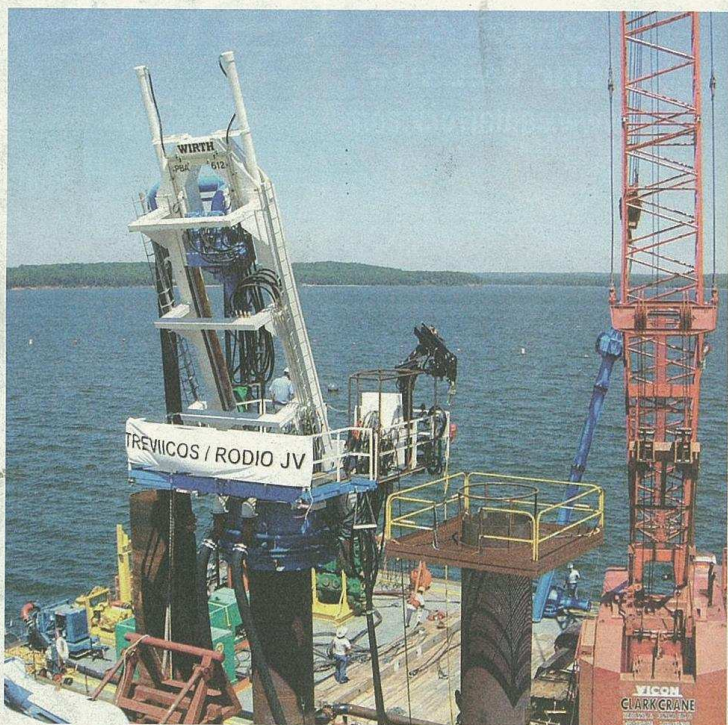
WIRTH rigs are being used for the foundation remediation.
