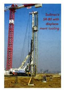
Moreover, since the drilling rig is utilised during drilling and extraction, it is operating more efficiently and productively than rigs used to construct conventional DDPs. Consequently, a smaller drilling rig can be used to achieve a comparably sized DDP.
