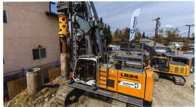
Doublestar drilling completing a segmental casing project in Calgary
