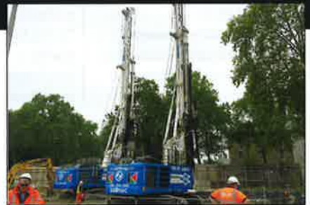
Keltbray's SR-75s at work on the Chelsea Barracks in London
