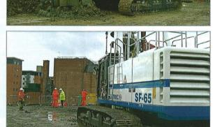
diameter piles of up to 24m length with multiple working platform. [This] made the working areas very tight and meant the 360° working ability of the rig was highly effective for the relatively confined spaces".
