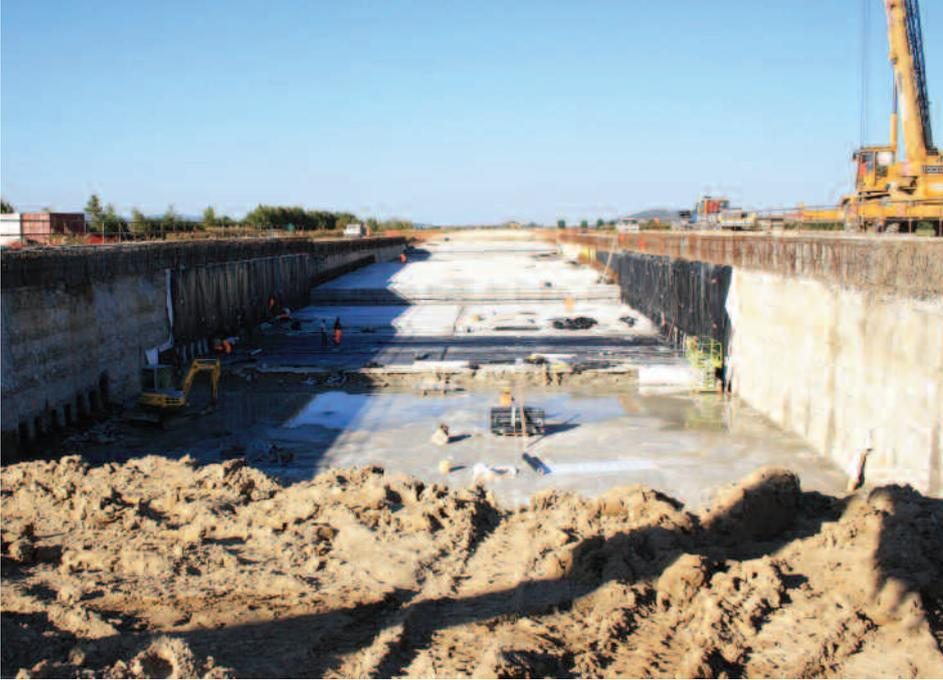
having a thickness of 1,000mm and 1,500mm, and a width of 2,500mm. The panels will be at depths of between 33.6 and 38.5m.
