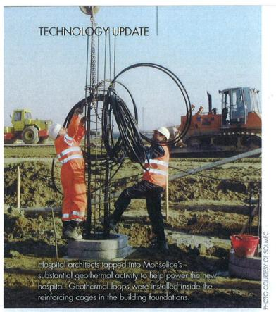
Crews used the SR-80 rig to dig 40 km of 600-mm diameter displacement piles to a depth ranging from 17 m to 24 m. After concreting the displacement piles in the foundation, crews pushed in a geothermal loop inside the reinforced cage.
