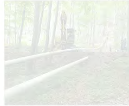
Welded cups pushed towards borehole
